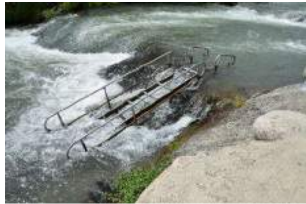
Figure 20 : steel stair for the athletes
