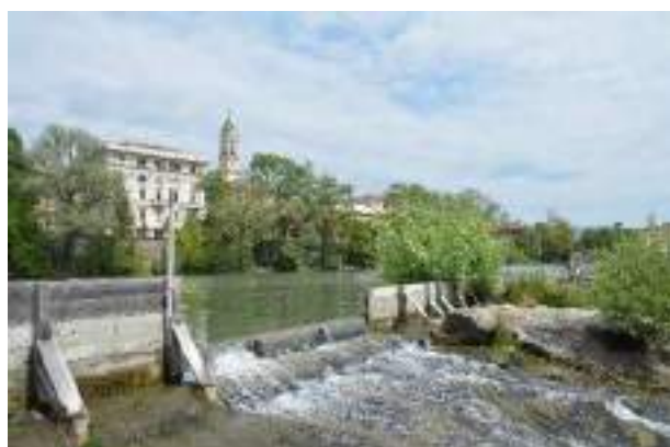
Figure 21: opening in embankment river
