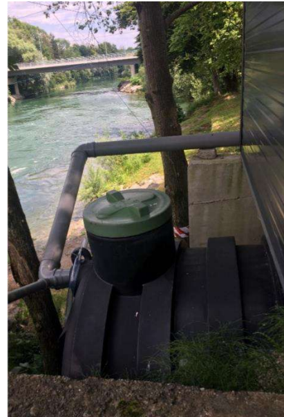
Figure 28 – Septic plastic tank below the toilette container
