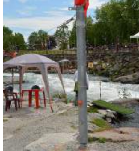
Figure 18: detail of fixed steel pole and cables
