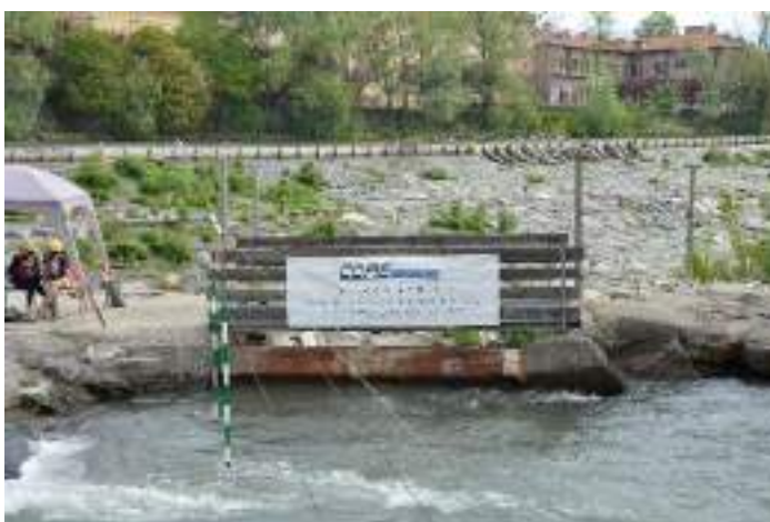
Figure 16: steel and wood crossing bridge
