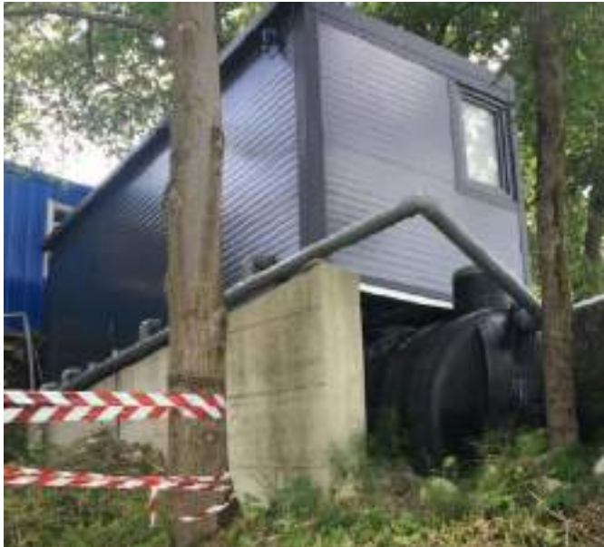
Figure 28 – Septic plastic tank below the toilette container
