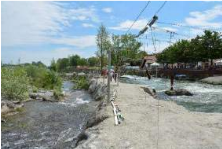
Figure 17: artificial rocks and concrete channel embankment
