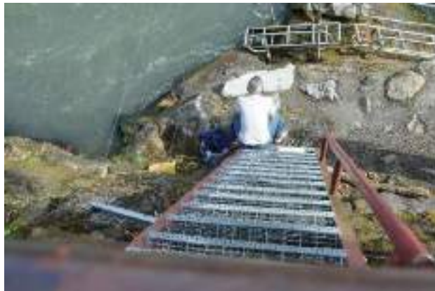
Figure 19 : steel stair to access the river
