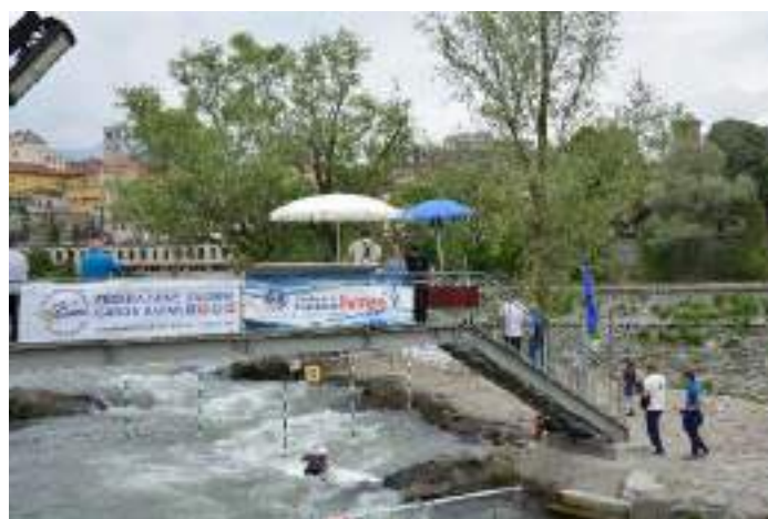
Figure 15: steel crossing bridge
