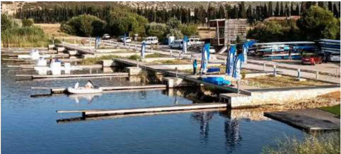
Figure 21: wooden pontoon at the start
